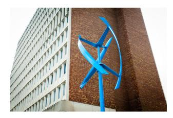
ISU has a vertical shaft UGE wind turbine located between the Sycamore Towers. This type of design allows the generator and gearbox to be located close to the ground so service and repair can be easy. This project was entirely experiential learning-based and integrated into course work for students. There are solar panels located on campus, but they are located on the sustainability campus. The Garden House and the solar sycamore design have solar panels.
